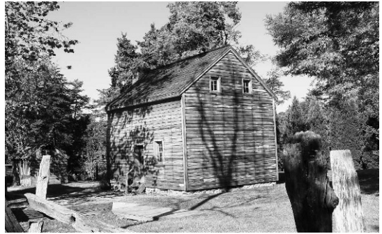
Figure 1. The Joseph Hoskins House, located at Tannenbaum Historic Park, Greensboro, North Carolina. The log structure was currently covered with clapboard siding. The house was believed to date to the Revolutionary War period ( ca. 1781), but earlier archaeological testing suggested a later date of construction (Stine 2005).
