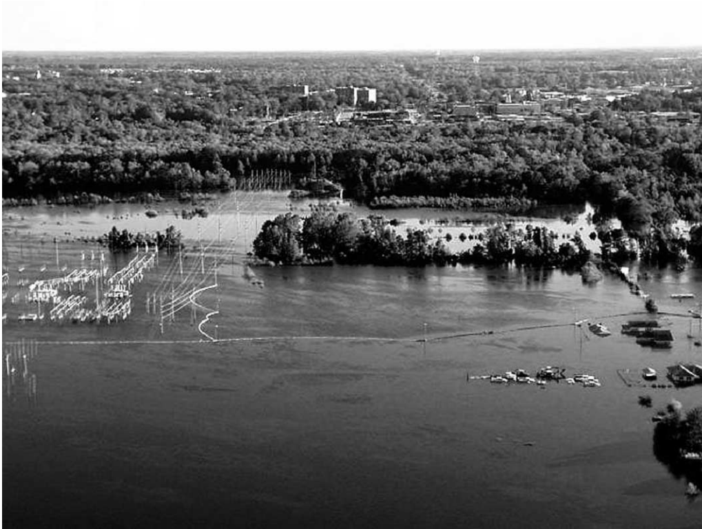
Fig. 1. Flooding along the Tar River in Greenville. View is towards the south with the power substation seen here on the left surrounded by booms. The Tar River channel is hidden behind the trees but downtown Greenville and the East Carolina University Campus dormitories can be seen on the far side of the river. (Source: Pitt County Management Information Systems).
