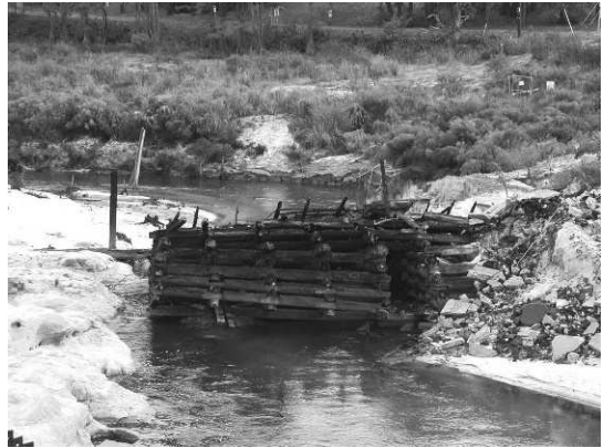
Figure 1. The Hope Mills crib dam in Little Rockfish Creek, North Carolina, after Hope Mills Lake drained and revealed the earthen dam (visible to the right) in May, 2003.
