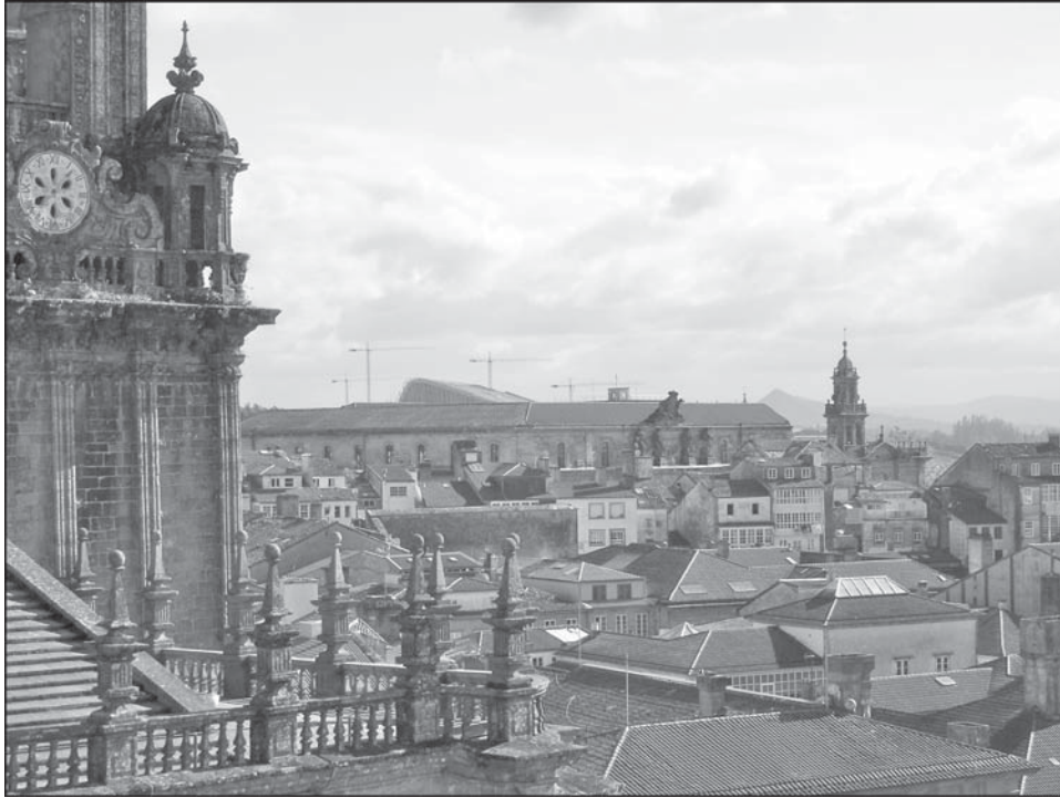
FIG. 4—The curved roofline and construction cranes of the looming Cidade da Cultura can be glimpsed from Santiago de Compostela’s iconic cathedral. (Photograph by the author, December 2008)
